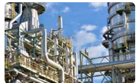
Kraftwerksbau | Power plant construction
