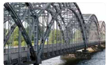
Stahlindustrie | Steel industry
